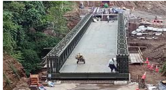
PCC & Abutment Reinf. installation
