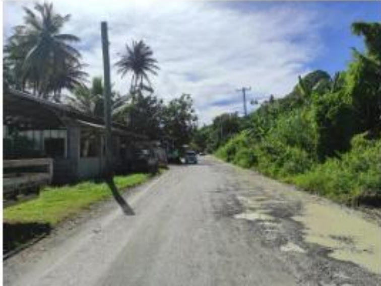
Figure 8.1: Existing Roadway considered for improvement under PRIME projects
