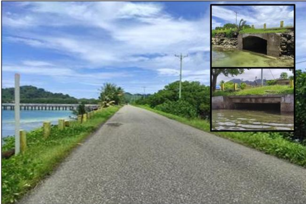
Figure 1.1: Lelu Causeway for improvement in Kosrae
