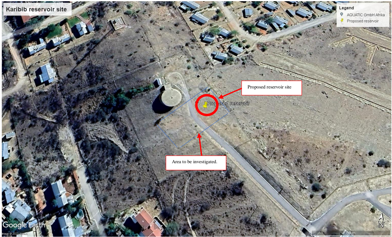
Figure 1 Aerial view of the Karibib NamWater Premises and Proposed Reservoir Location (GPS coordinates lat: -21.939448°, lon: 15.859182°).
